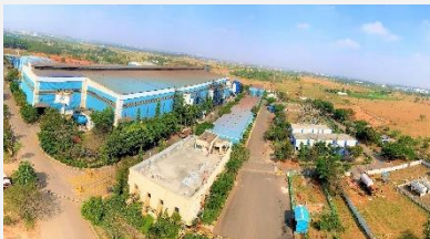
Utilizing wind power and solar power
