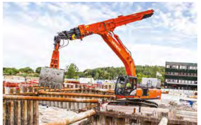
Special application excavators
