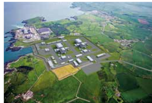
Power systems and equipment
