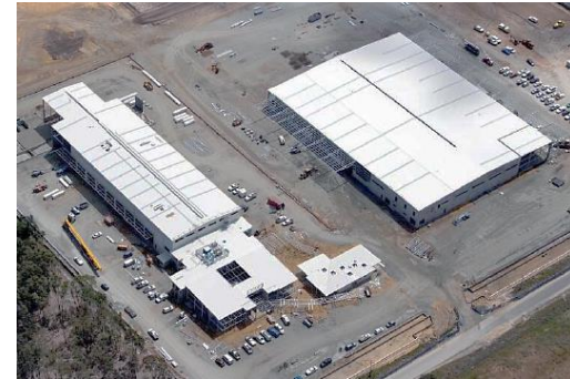
The new Perth branch under construction
