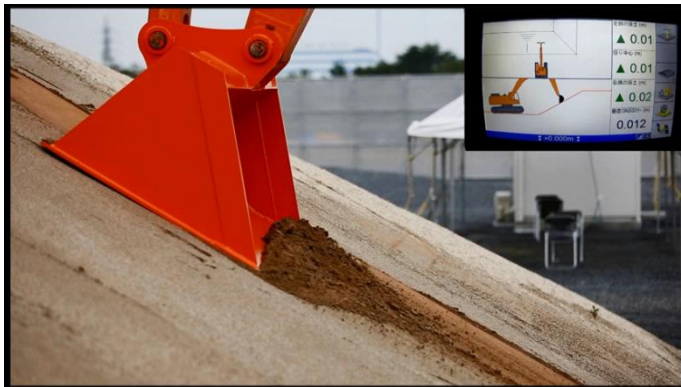
Slope work by semi-automated excavator
