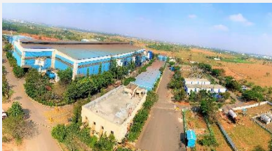
Utilizing wind power and solar power
