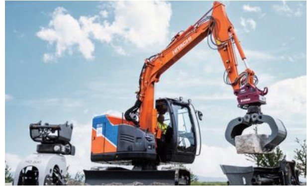
Battery-powered excavator (8-ton class) working at a construction site
