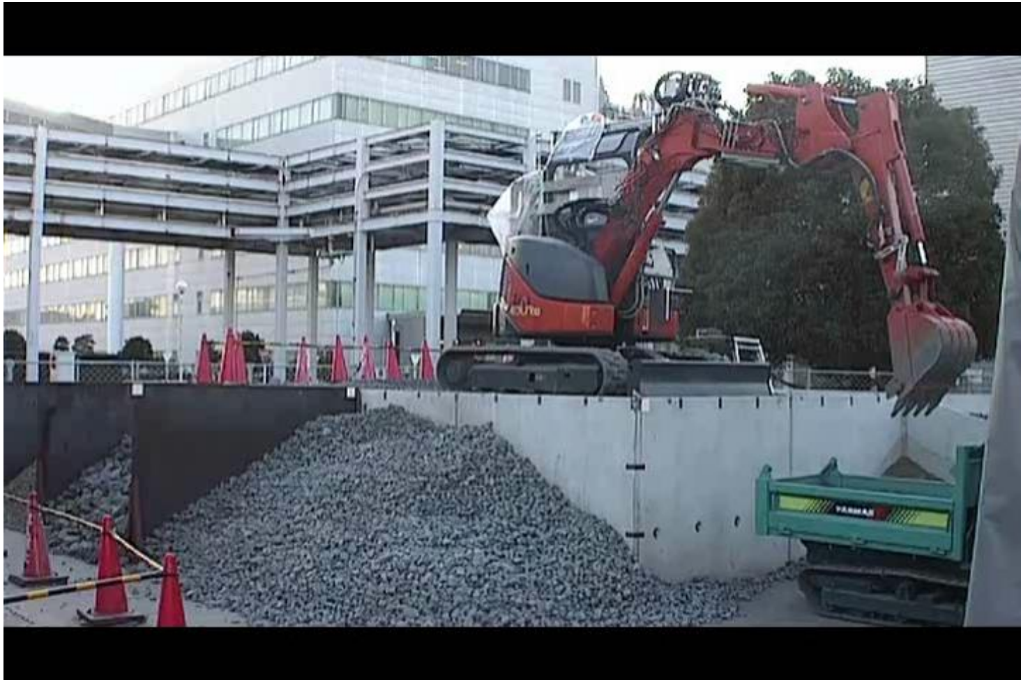
Mini excavator automatic excavation and loading tests
