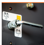
Battery disconnect switch
