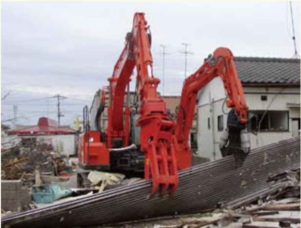
Twin-arm machinery operating in Ishinomaki We developed this product under contract from New Energy and Industrial Technology Development Organization (NEDO).
