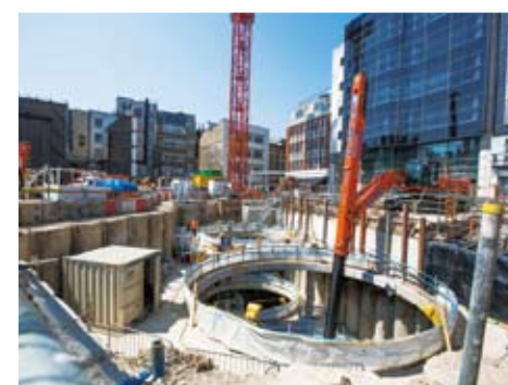
ZX350LC excavator with telescopic arm and clamshell bucket in operation excavating a tunnel for the London Underground
