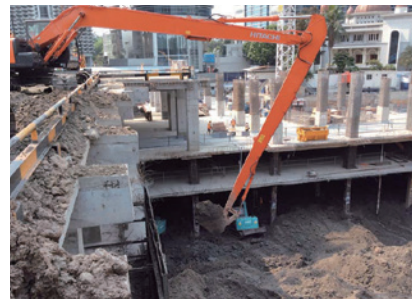
Scooping up underground earth and sand from an above ground position. Pictured is the ZX210LC-5G (18-meter front) operated in Indonesia.
