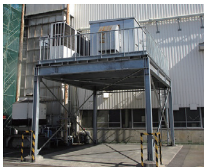
Unit for reusing the waste heat of Tsuchiura Works inside the plant's air conditioning system
