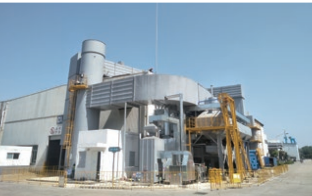
VOC gas cleaning and deodorizing system at Hitachi Construction Machinery (China)
