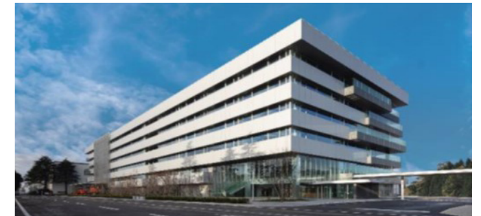
Exterior view of a recently constructed engineering building (Tsuchiura City, Ibaraki Prefecture)
