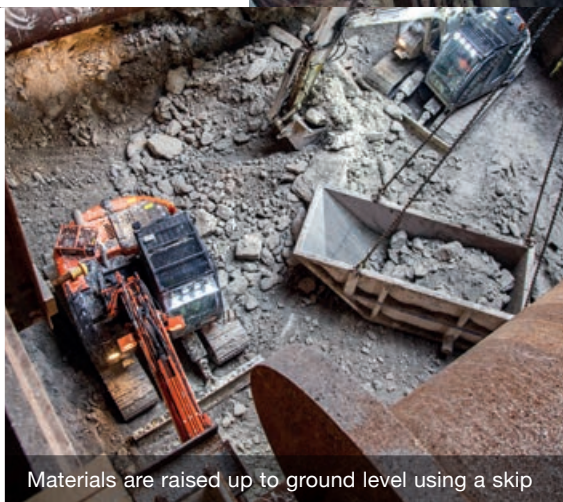
One of three Cityringen shafts under construction
