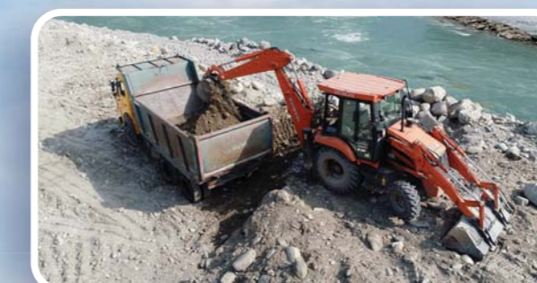
RIVER BOULDER CLEARING
