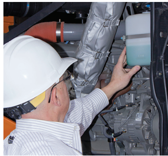
Coolant Tank Reservoir Inspection
