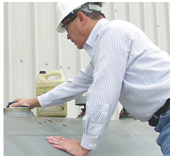
Adding conditioner to fuel storage tank
