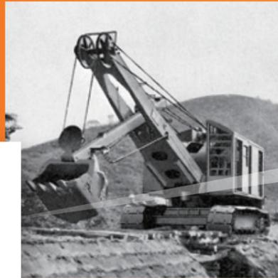
The U05, Hitachi's first cable-operated power shovel developed in 1949. Began mass producing and selling the U06, the successor machine to the U05, in 1950. It was called an all-purpose excavator, which acted as a powerful driver behind Japan's efforts to restore its national infrastructure following World War II. (Pictured is the U05)
